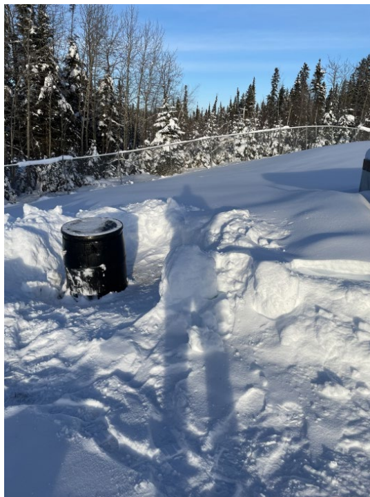
Photo 3: Manhole downstream of effluent chamber prior to environmental discharge
