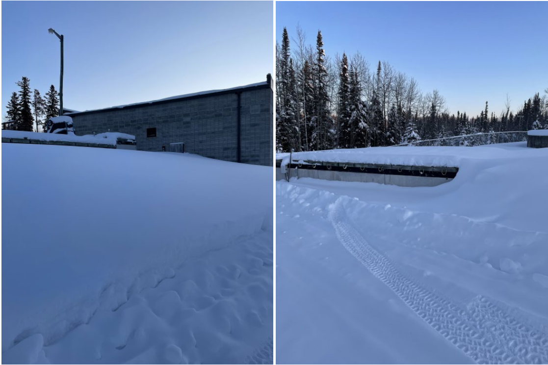
Photos 2A (left) & 2B (right): Rear of Service Building with adjacent effluent chamber (inlet-side) & same adjacent effluent chamber outlet-side
