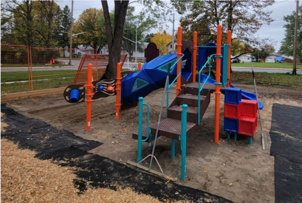
Image 9: New small play structure (installation phase), Fort Frances, 2023
